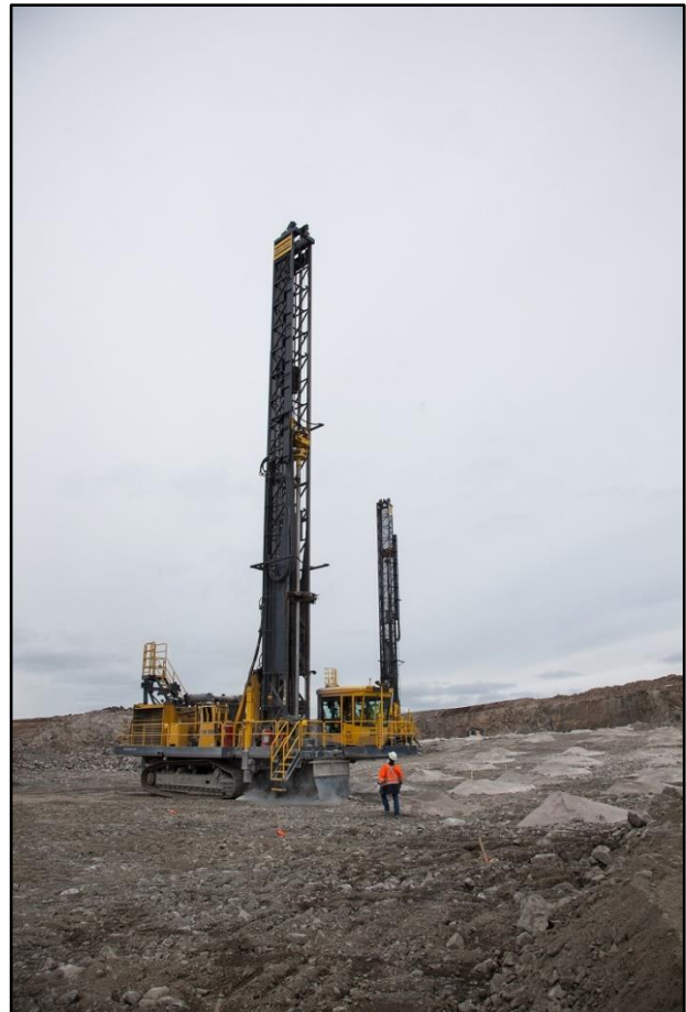
Drilling in the Gahcho Kué Mine open pit
